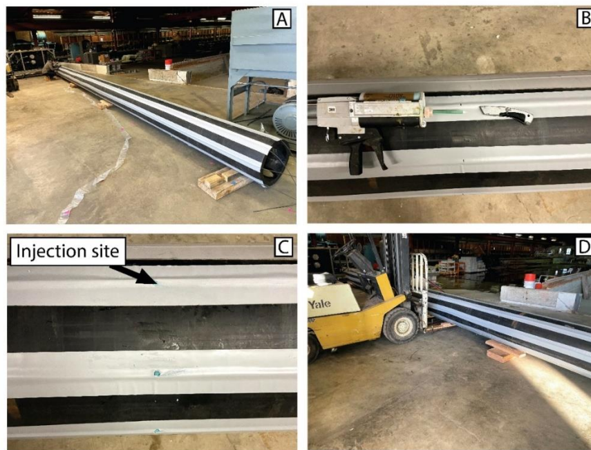
Figure 3. Images from a bending test at UC Berkeley's Richmond Field Station. A) fully instrumented pipe before bending; B) epoxy injection process; C) final appearance after injection; D) forklift bending pipe by lifting at center
